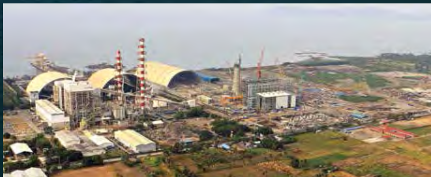
Construction of the 2x150 MW CFB power plant in progress. Target commissioning of both units is H1 2015.
